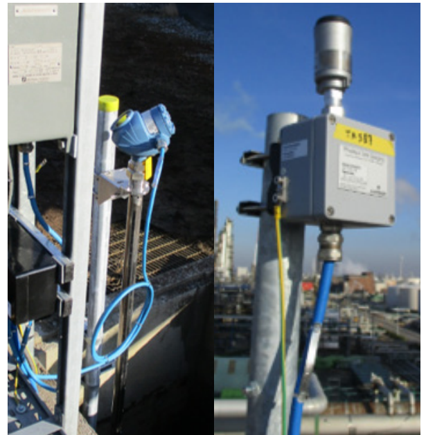
Rosemount 5300 Level Transmitter and Emerson 775 THUM Adapter installation installed on drain pit for early detection of potential hydrocarbon leaks
